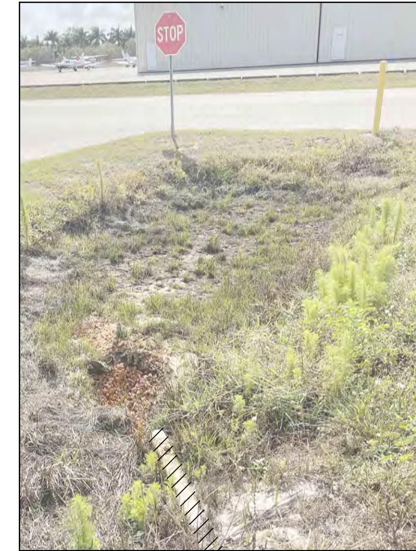
CONTRACTOR SHALL DEMO THE COMPLETE (E) U/G OWS DISCHARGE PIPE
