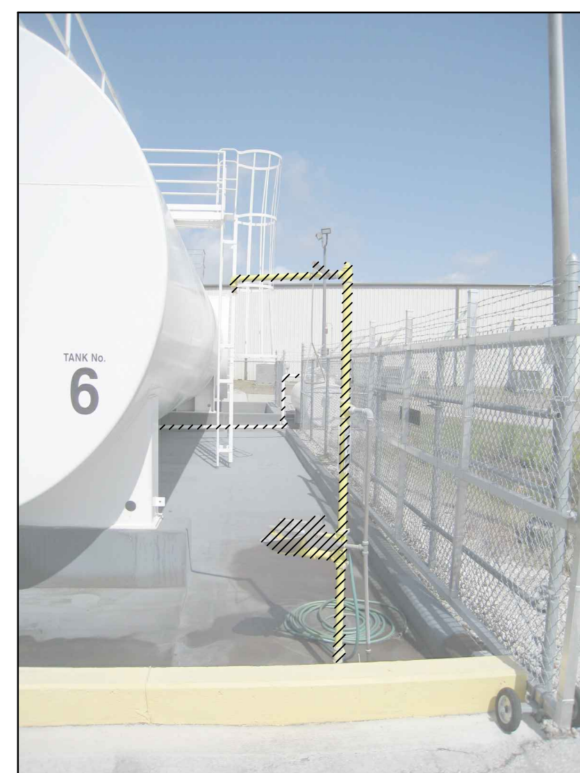
T (E) EYEWASH STATION AT TANK #6 SCALE: N/A
